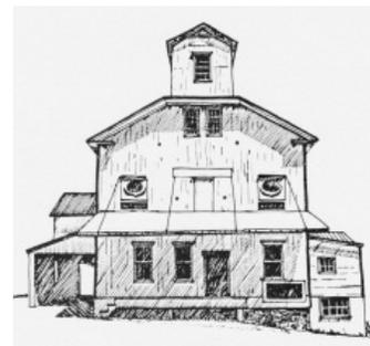
The feed mill was built by the Doering brothers in 1856. The original two and half storey section at the back was enlarged around 1910 with the addition of the third storey and the entire front portion. The structure is made of massive timbers, held
